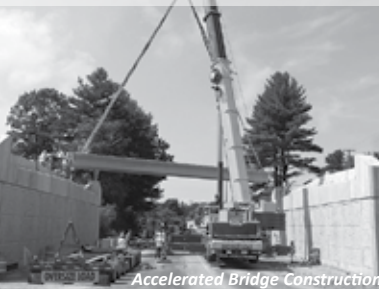
Accelerated Bridge Construction
