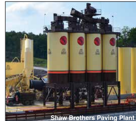
Shaw Brothers Paving Plant
