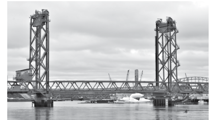
Researchers are monitoring a variety of variables on the Memorial Bridge, including structural performance, weather and tidal currents.
