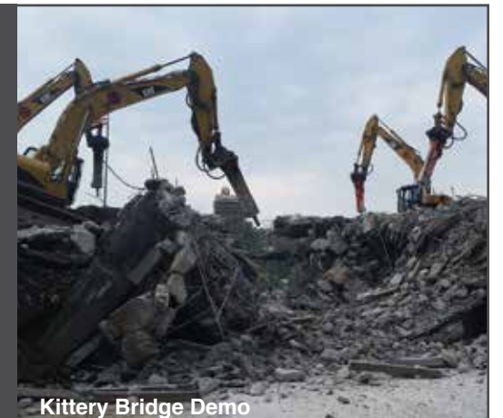
Kittery Bridge Demo
