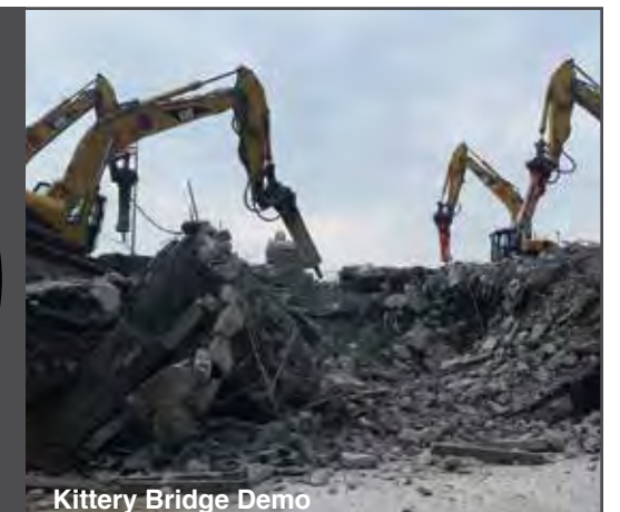
Kittery Bridge Demo
