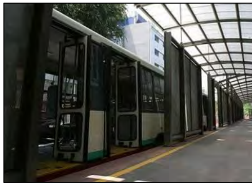
Typical Level Boarding Platform proposed at Major and at several Minor Stations (Source: Mexico City MetroBús)
