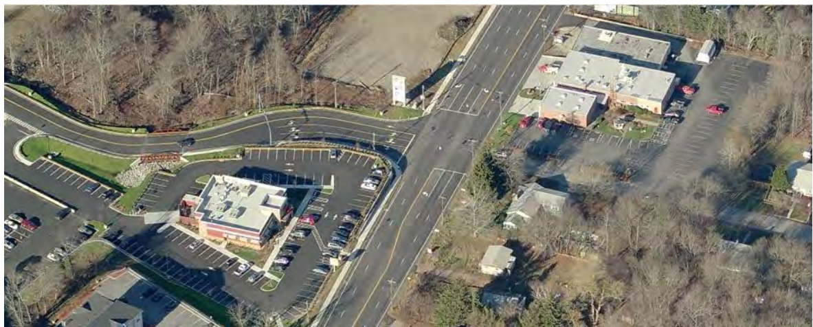
Route 32 Traffic Lane Improvements
