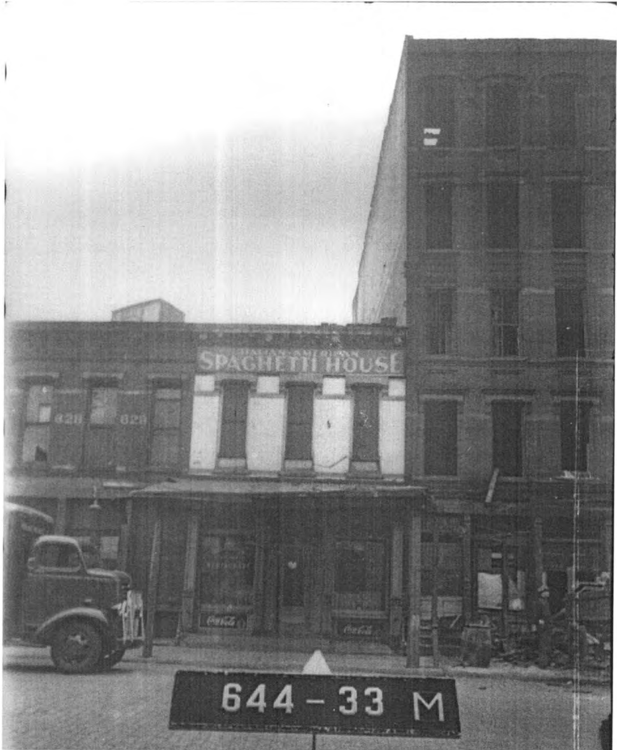
823-825 and 817-821 Washington Street Source: Department of Taxes (c. 1939) Photo: NYC Municipal Archives
