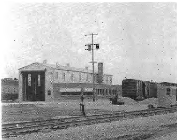
Above: Southwesterly view of the yard, showing the diesel house in the center, with car repair tracks at left and classification tracks beyond. At the right are storage tanks for sand and diesel fuel oil.
