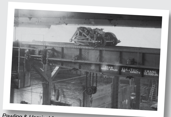
Pawling & Harnischfeger worked with crane specialist A.J. Shaw to rebuild a failed overhead crane on behalf of the Edward P. Allis Manufacturing Company in 1888. Soon after, manufacturing firms began to clamor for more such cranes designed and built by Pawling & Harnischfeger. Suddenly, the firm had a product line all its own.
