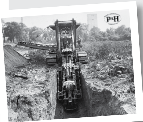
A P&H® 152 ladder-type trenching machine circa 1915 quickly claws a pipeline trench through the earth in what is today the southeast parking lot of the P&H Mining Equipment factory in West Milwaukee.
