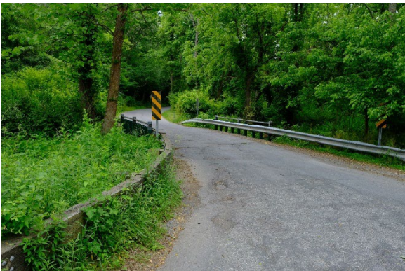
Narrow bridge crossing over the Hights Branch
