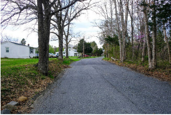
Looking north at the paved section of Hoyles Mill Road
