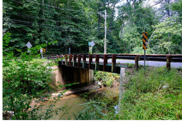
One-lane bridge over the Watts Branch
