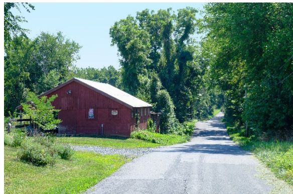
Stable close to Hughes Road
