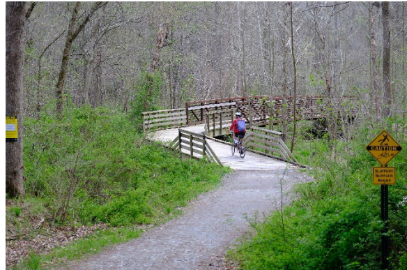
Bridge crossing over Little Seneca Creek
