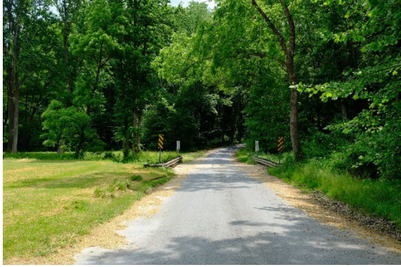
Bridge crossing the Hights Branch
