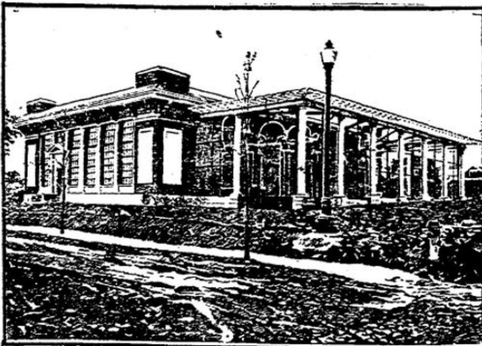
AT 61ST AND FOREST, VINES GROWING ON A WIRE SCREEN BETWEEN THE PERGOLA COLUMNS WILL SOON HIDE THE TRANSFORMERS
