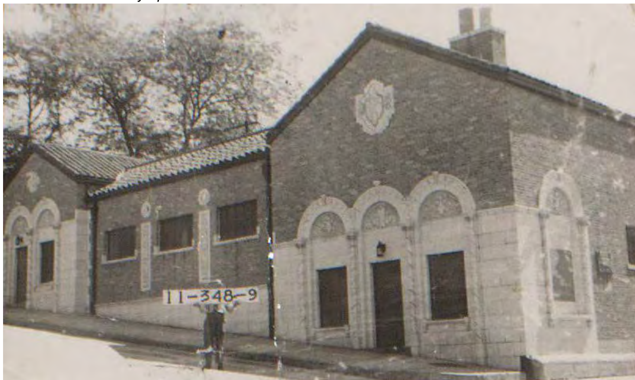
Figure 16. Substation H (constructed 1931), 4600 block of Broadway, 1940 Tax Assessor photograph. Source: Missouri Valley Special Collections.
