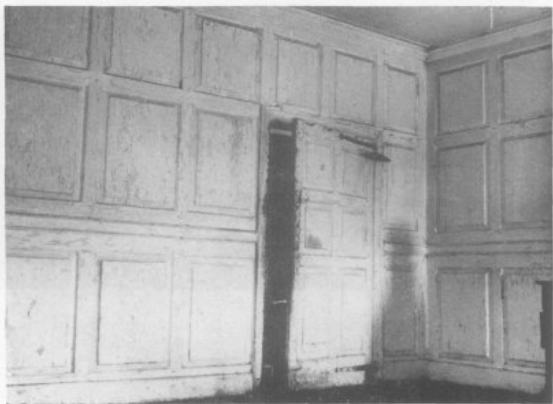
The rare transitional panelling at Genesar has small squares and near-squares, and a door with a double-cross design. All this woodwork has disappeared. Author's photograph, ca. 1934.
