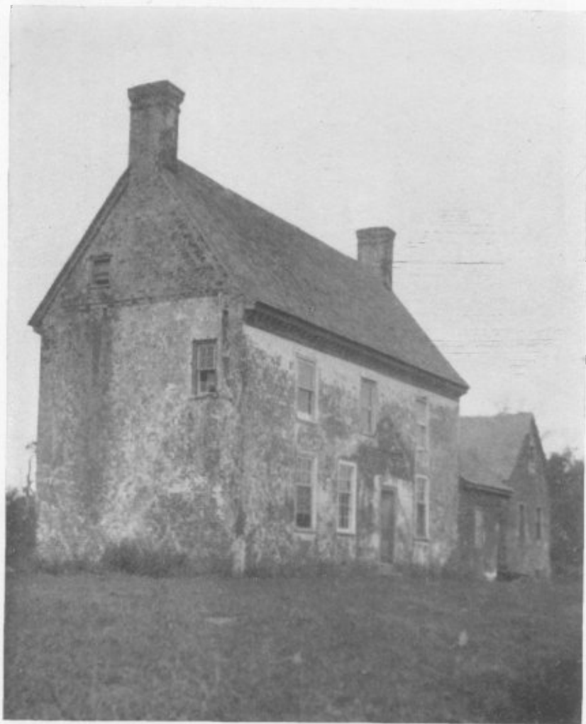
The west gable-end of Genesar in which lozengy may be seen by keen eyes, is marked by strong Gothic verticality. Author's photograph, 1934.
