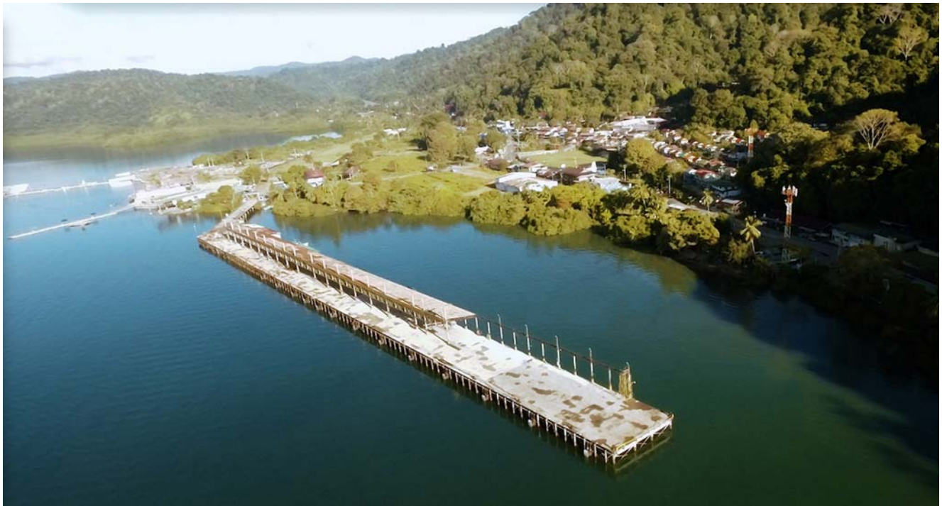
Golfito Main Wharf
