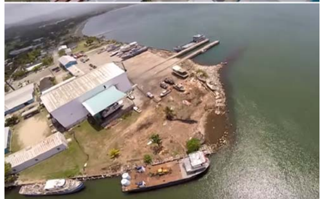
Puerto Cortes Naval Port Piers W of Isla Santa Margarita
