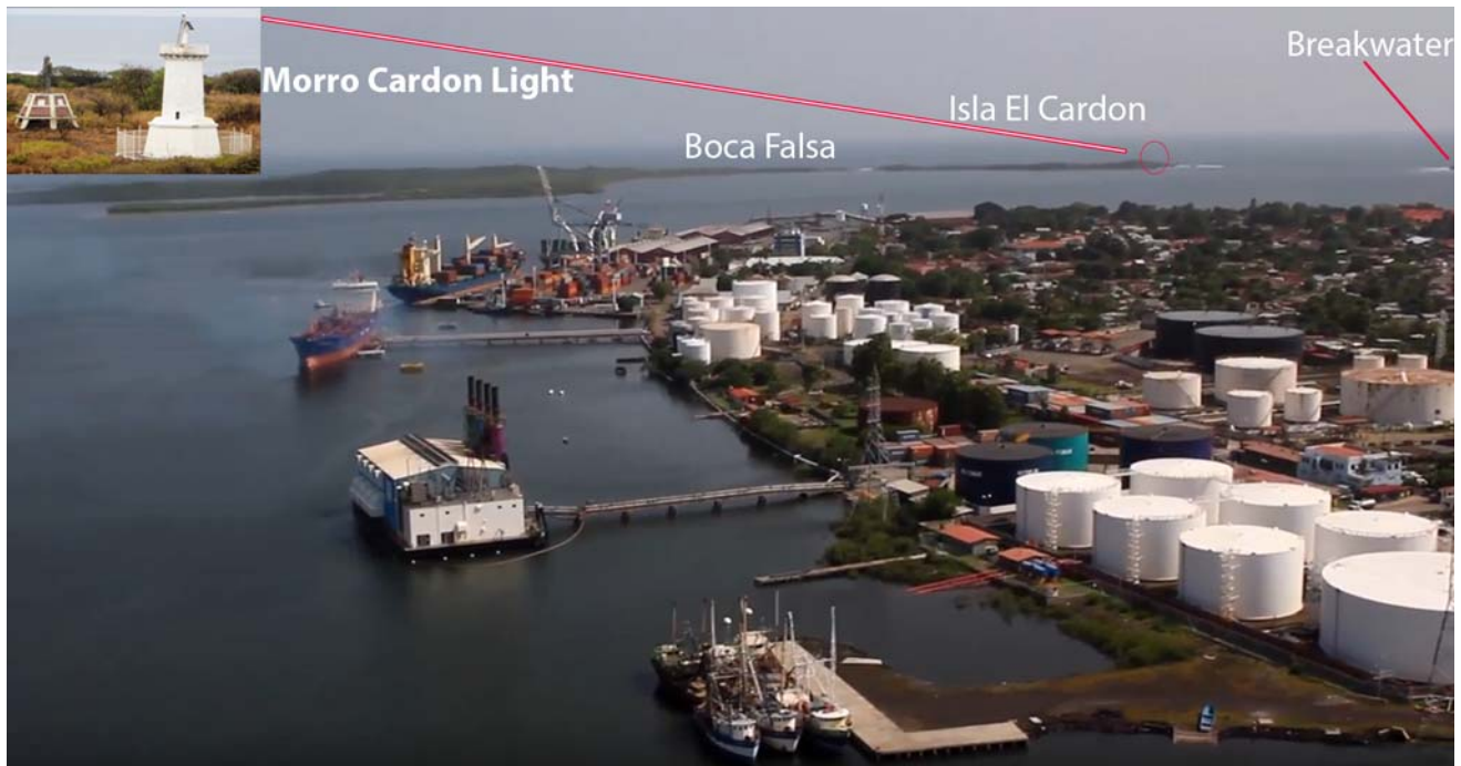
Puerto Corinto berths and approach channel between Isla El Cardon and breakwater
