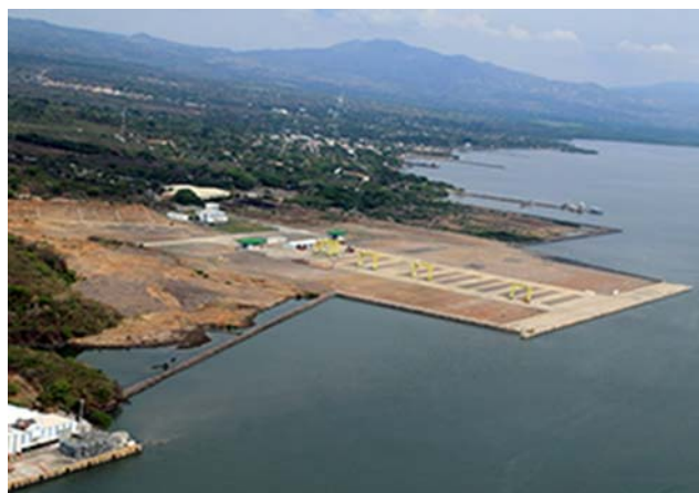
Puerto La Union Wharf from SE
