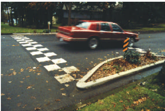
FIGURE V-17. TYPE 3 OBJECT MARKERS ON CURB EXTENSIONS AND EDGE ISLANDS
