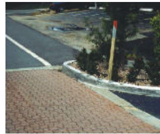
FIGURE V-20. ADDITION OF LANDSCAPING ON A PROBLEM CHOKER PREVIOUSLY MARKED WITH REFLECTIVE POST ONLY
