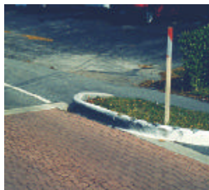
FIGURE V-20. ADDITION OF LANDSCAPING ON A PROBLEM CHOKER PREVIOUSLY MARKED WITH REFLECTIVE POST ONLY
