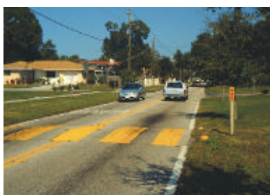
FIGURE V-7. OBJECT MARKER NEXT TO SPEED HUMP ON A CURBKESS SECTION
