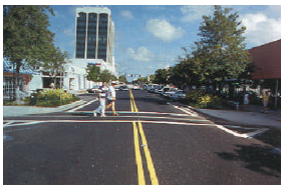
FIGURE V-19. NO MARKINGS REQUIRED WITH PROTECTED PARKING BAYS
