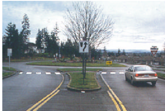
FIGURE V-16. SIGNING OF ROUNDABOUTS
