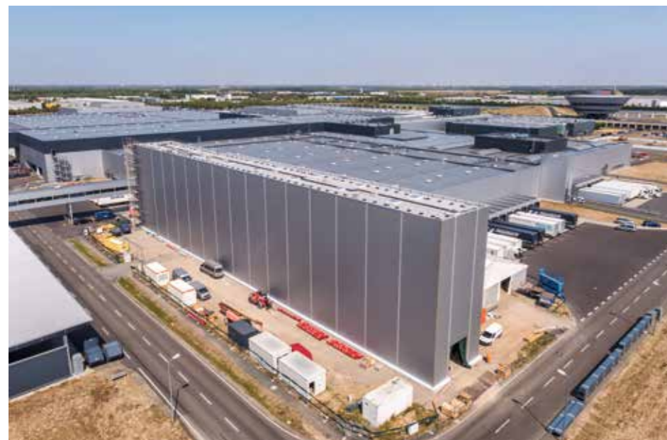
AUTOMATED SMALL-PARTS STORAGE SYSTEM
