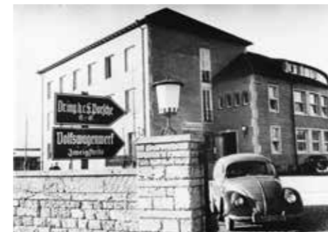
BRICK BUILDING, THE CURRENT-DAY PLANT 1
