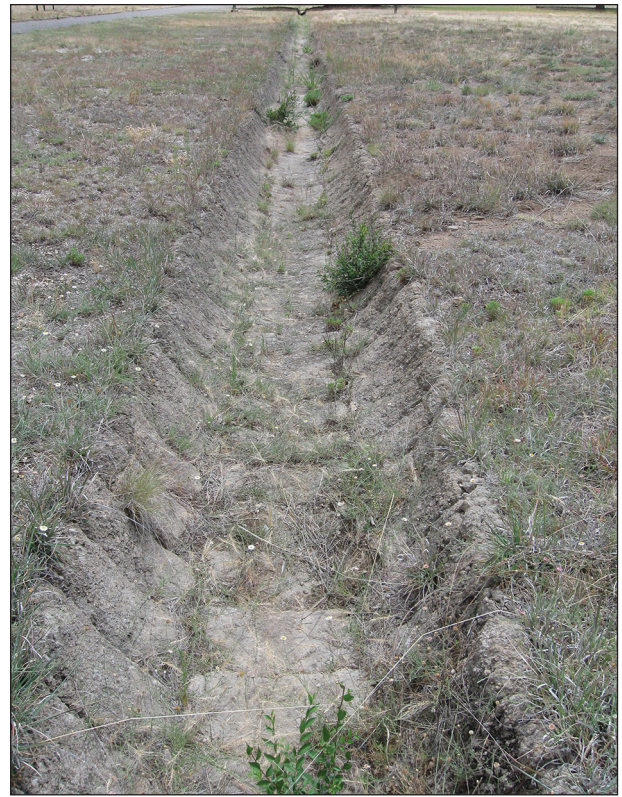
Figure 5.4. WPA drainage ditch that extends along the eastern border of the hospital grounds.
