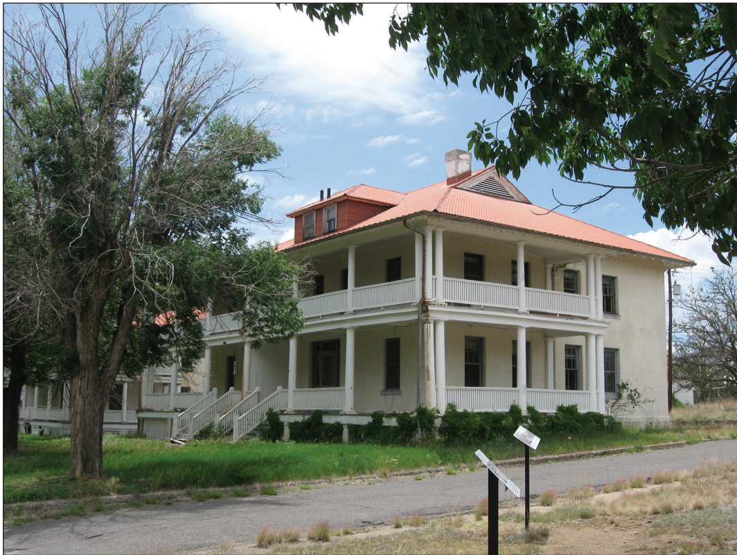
Figure 4.3. Officers' quarters at Fort Bayard, view southeast. This building was constructed in 1877.
