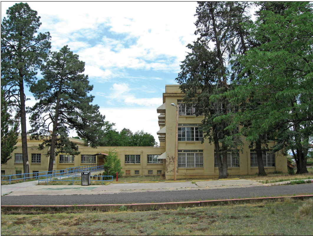
Figure 8.1. LA 3546, U.S. Veterans Hospital No. 55 at Fort Bayard, view south.
