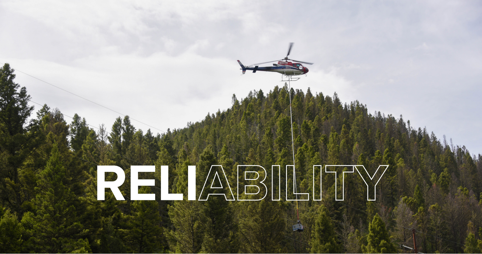
▲ NorthWestern Energy uses aerial tree trimming along some of our transmission lines as part of our Wildfire Mitigation Plan.
