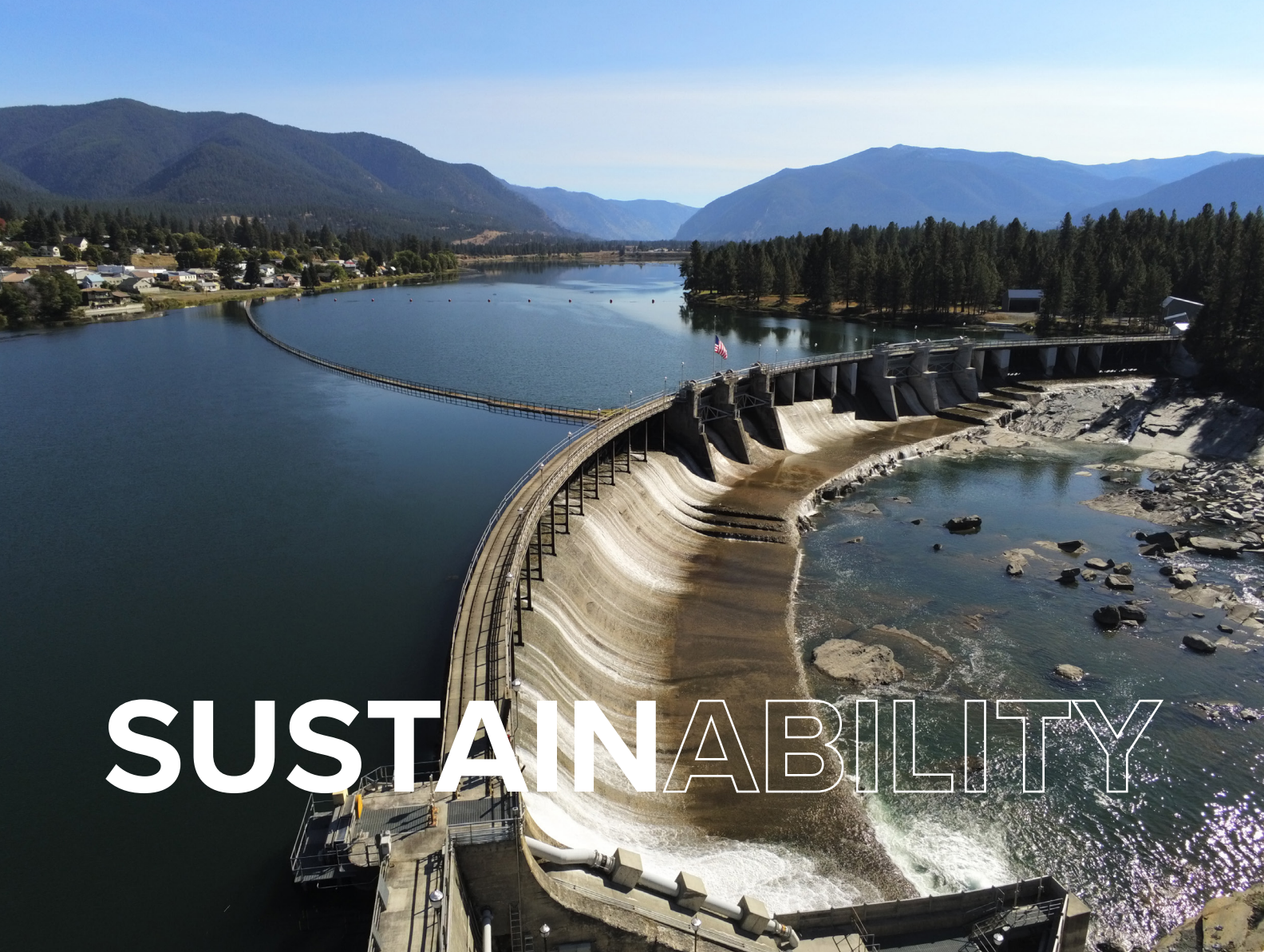
▲ Thompson Falls Dam in northwest Montana is a 94-megawatt facility. We are proud of our diverse generation fleet of hydro, wind, natural gas and coal resources.
