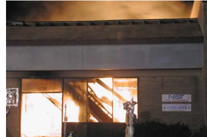
Roof collapses in shopping center store fire.
