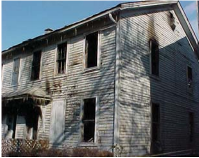
Front view of the Iowa duplex home.
