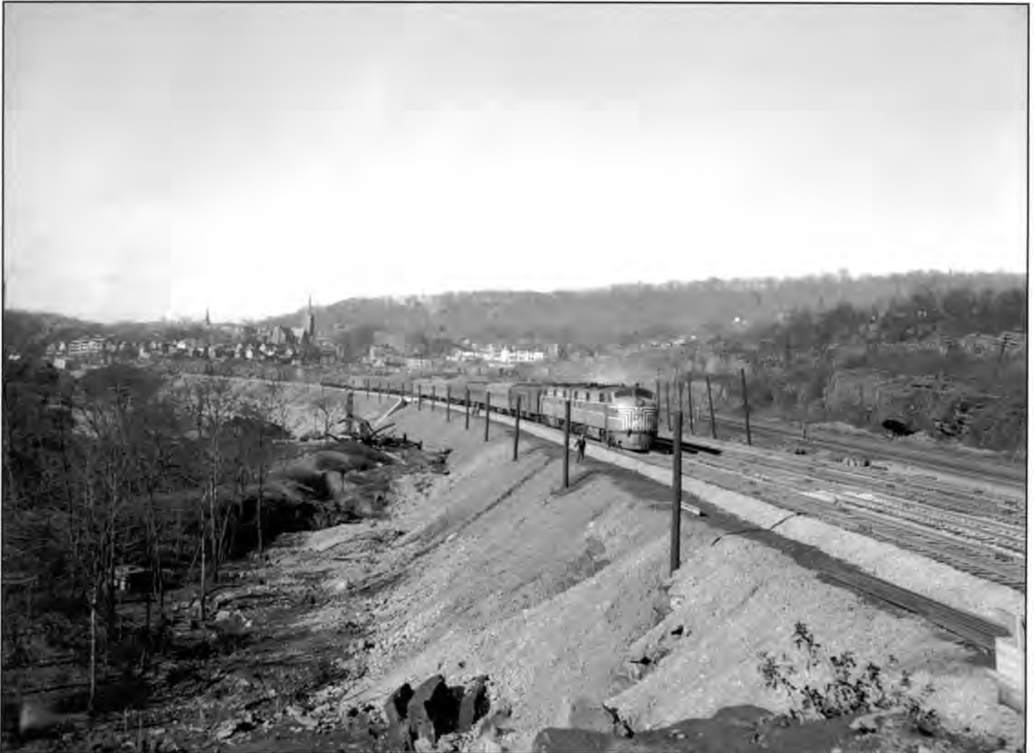
E7 4001 and an unidentified mate traverse the new Gulf Curve alignment with a secondary train on November 9, 1947. The photo shows the scope of the project. Note the old alignment, as indicated by the pole line at the extreme right in this photo. Negative 7941-8.
