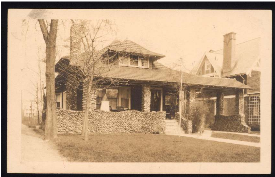
Figure 2.6: The Weeber house at 106 Manning Boulevard in Albany, c.1915. Marion Weeber wrote the house was designed and built by her father. NYSM Collection, H-1987.39.2.
