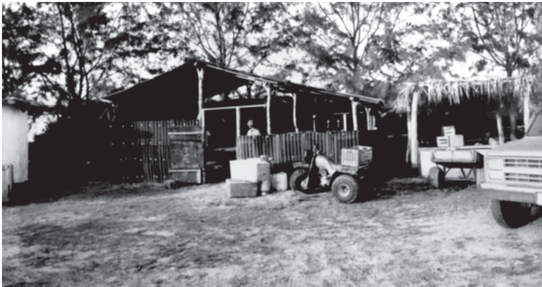
The Rancho Nuevo kitchen in 1978 (Photo: P. Burchfield).
