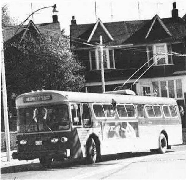
Toronto began the modern trolley bus era in North America in the late 1960s by buying unpowered Flyer buses and installing rehabilitated electrical gear in its own shops (photograph by J.P. Aurelius).
