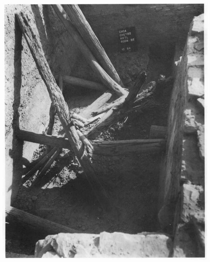
Fig. E.4. Remains of ceilings, Room 92. The viga found in place is horizontal at center.
