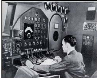
Above caption: "At this big panel, the flight engineer controls the motors. The door at right leads to a motor-inspection passageway."
