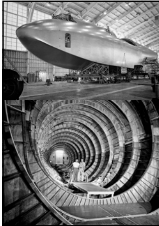
Top: caption: "This is the hull of the Hughes Hercules, called by its builders the largest plane in the world, in construction at the Hughes Aircraft Co. plant at Culver City. The hull is 220-feet long, 30-feet high and 24-feet wide (July 1945)."
