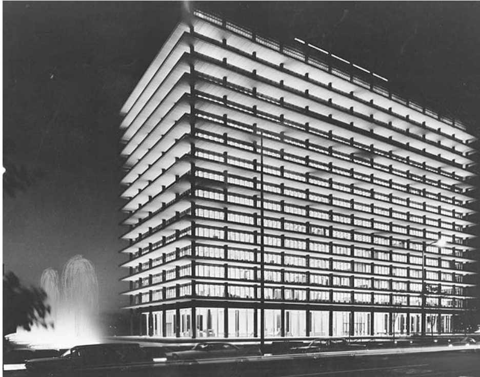
DWP General Office Building, 1964 L.A. Historic-Cultural Monument No. 1022 (Los Angeles Public Library)
