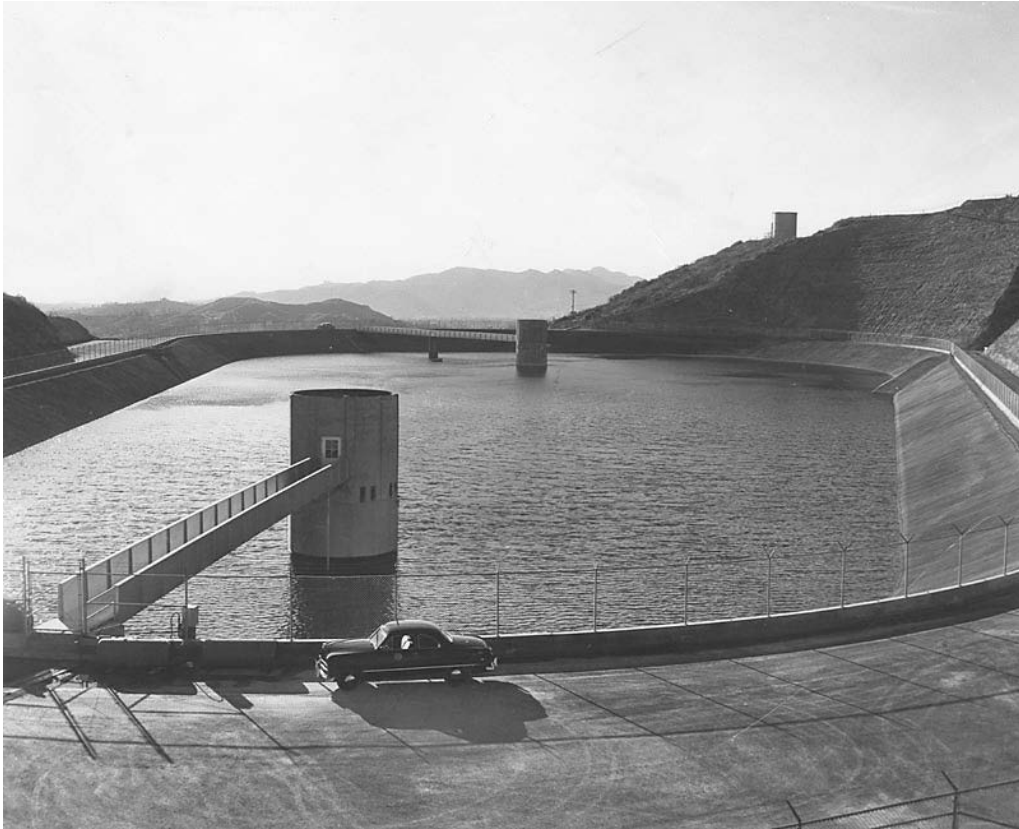
Eagle Rock Reservoir, 1952-1953 (Los Angeles Public Library)
