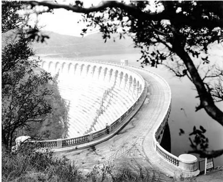
Mulholland Dam, 1923-1924, before fill and landscaping Los Angeles Historic-Cultural Monument No. 421 (Los Angeles Public Library)
