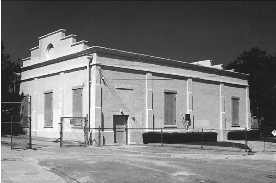
Garvanza Pumping Station, 1907 L.A. Historic-Cultural Monument No. 412 (L.A. Office of Historic Resources)
