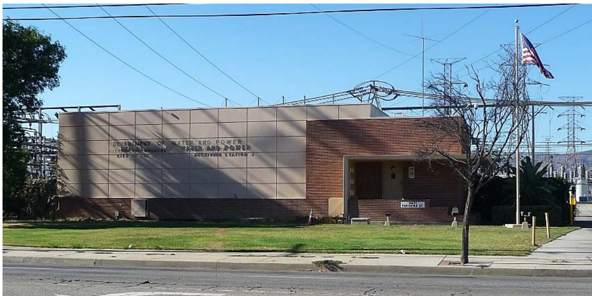
Receiving Station J, 1952 18821 West Parthenia Street, Northridge (SurveyLA)
