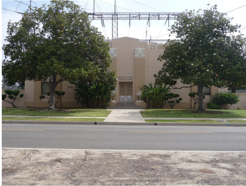
Control Building, Receiving Station E, 1938 Cahuenga Boulevard and Whitnall Highway, North Hollywood (Survey LA)
