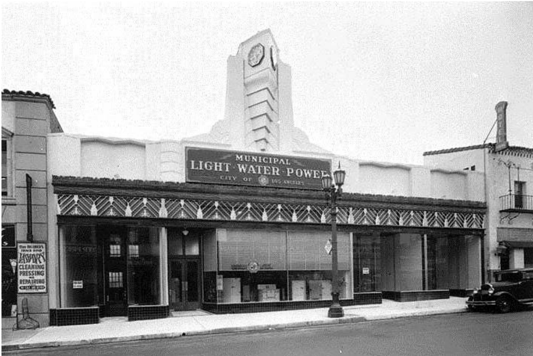
Branch Office, 1932 1613 Cahuenga Boulevard, Hollywood (Los Angeles Department of Water and Power)
