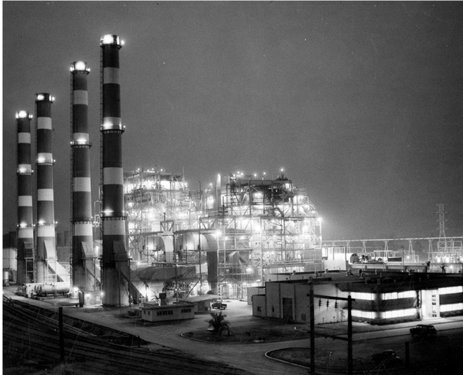
Valley Steam Generating Plant, 1951-1956
