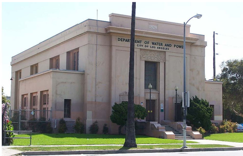
Distributing Station Number 4, 1928-1929 5716 South Figueroa Street, Southeast Los Angeles (SurveyLA)
