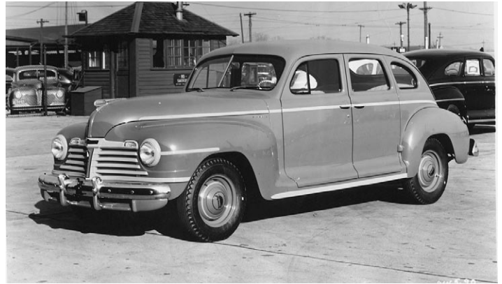
1942 Plymouth Special-Deluxe sedan (nc): black-out version. Note deleted and abbreviated fender mouldings, and painted trim and hub caps.
