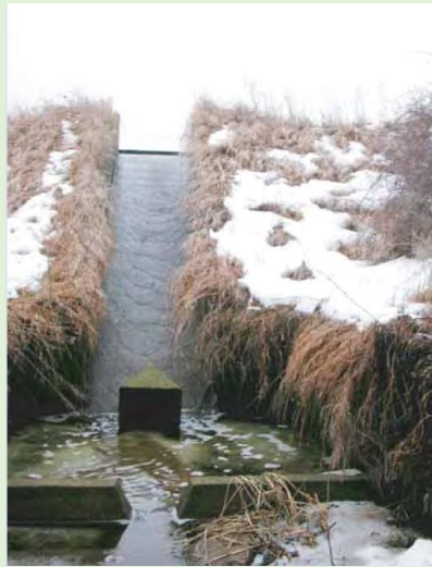
Spillway still works in 2020.
