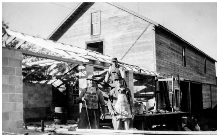
Garage being built in the late 1940s still stands today.
