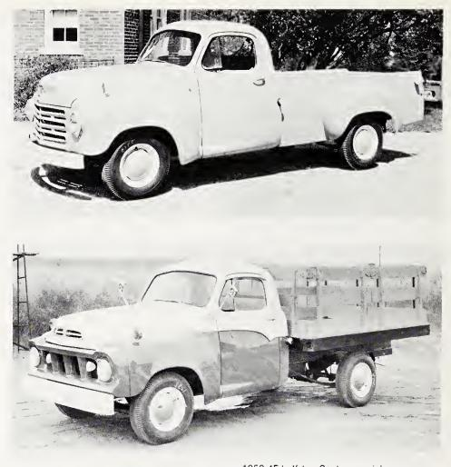
1959 4E half-ton Scotsman pickup. 1959 4E7-112 half-ton V-8 rack body.
