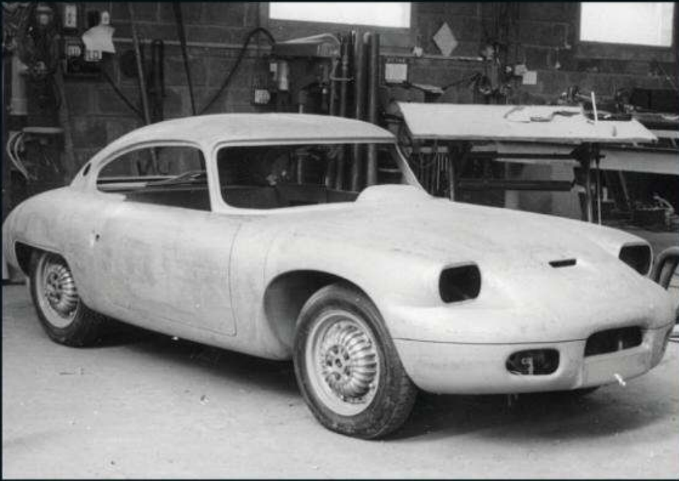
Panhard-CD prototype was steel, but production cars and Le Mans racers were glassfibre
