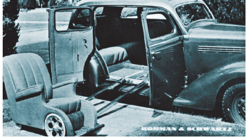
The chair had six wheels, two hidden here, and moved out of the car sideways. Aluminum U-section channels formed ramps. Hasps locked the chair to floor, and upholstery matched the car's interior.
