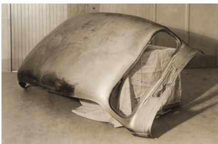
The Budd Company of Philadelphia did considerable work for Studebaker in the mid 1930s. Shown here in a photograph dated October 1935 are stamped body panels that were used on the 1936 Studebaker Dictator and President cars. This stamping was referred to by Budd as a "mono-roof."
