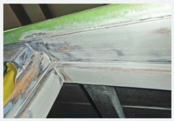
According to the restorer, rather than cut and replace the small damaged sections of exterior wood trim, the team cleaned the affected areas and sealed them with Durham's Rock Hard Water Putty, which is easy to mold and doesn't shrink while curing.
