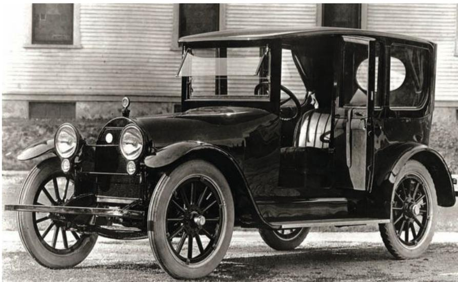
Kissel had a reputation for innovation in body design, and this 1918 Kissel “100-Point Six” series auto wears a striking “Staggered-Door” body. In this design there were two doors, one up front on the driver's side, and one in the rear on the passenger side.
