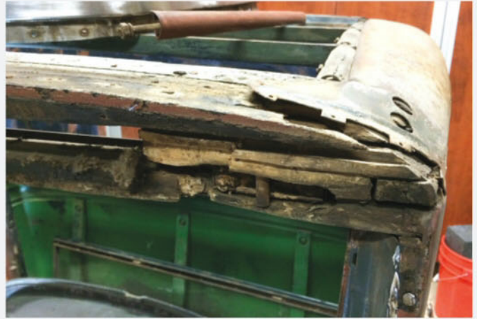
While the frame was being checked, focus shifted back to the cab. After removing the factory visor, a standard feature, it was discovered that a section of the wood framing—still employed to support the fabric top—had suffered the wrath of dry rot.
