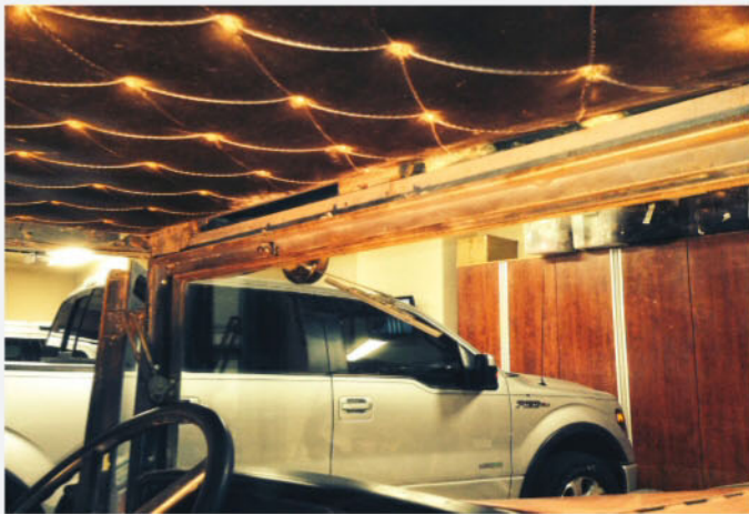
At the top of this image you'll see the diamond-pattern upholstery installed in Mexico decades prior. The pivot points and slide braces for the front windshield were functional, as was the wiper motor, but the wooden header above showed water stains.
