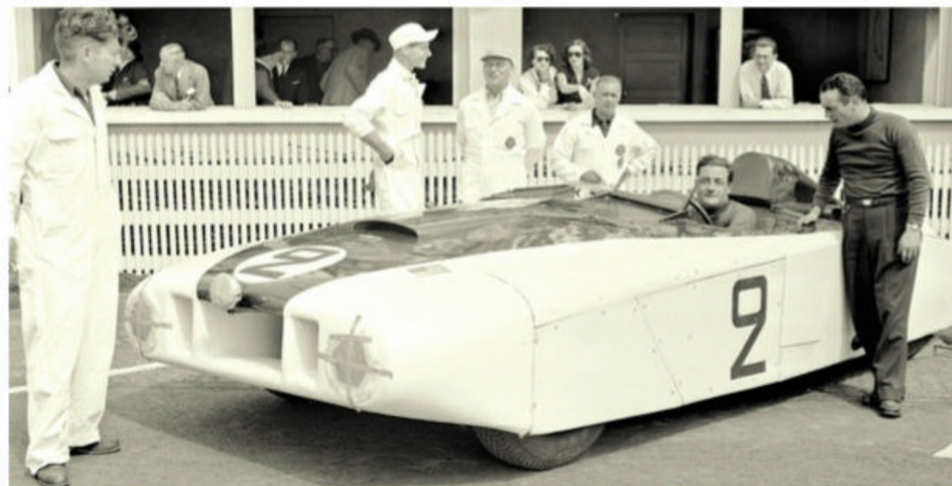
The second Cadillac, which French crowds called Le Monstre ("The Monster") was fitted with streamlined aluminum bodywork fashioned by moonlighting workers from Grumman Aircraft. It took 11th place.
