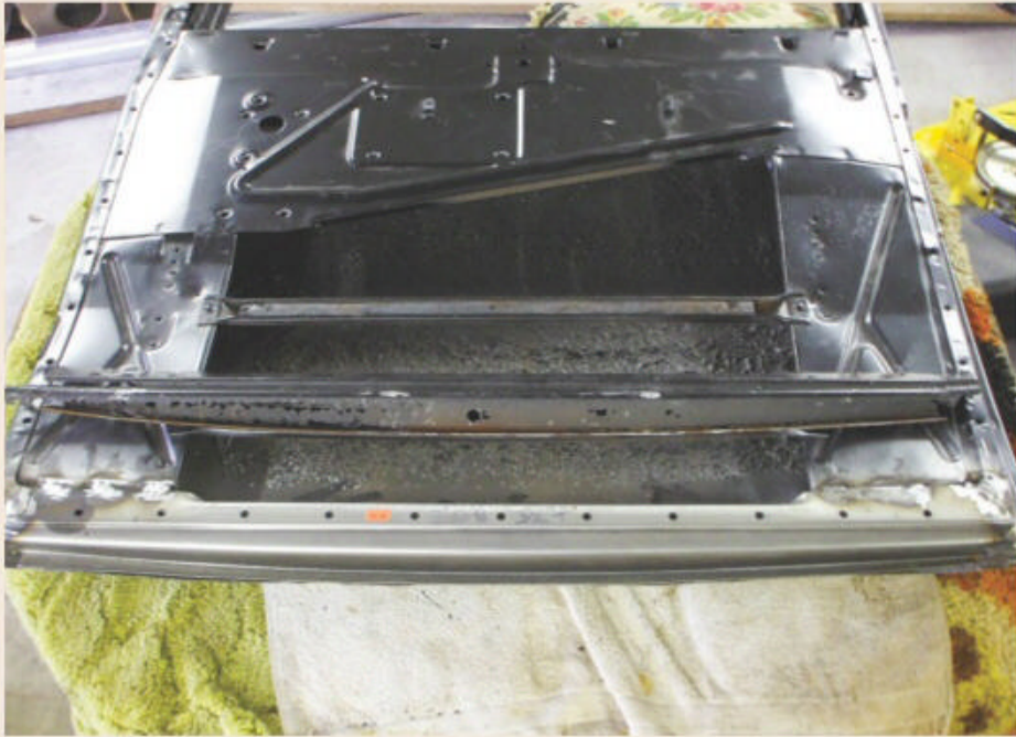
Both doors needed their lower portions completely repaired with new metal. Shown is the replacement piece welded in with the old cutout rusted section sitting on top for comparison.
