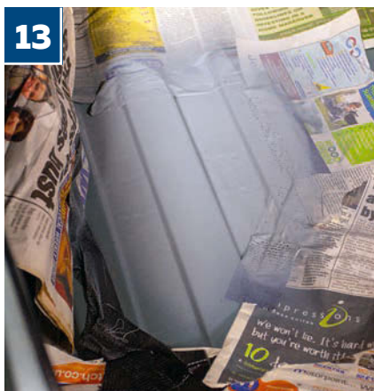
13 The problem was slight pitting on two lips of the floor's raised rails; isolated to a tiny area, there's no doubt the issue was superficial, but Dan reasoned it worth treating and painting in epoxy primer
