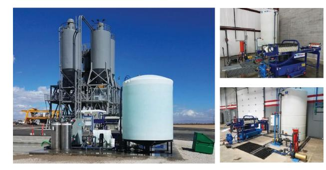
Water Treatment Solutions custom designs, installs, and services filter press-based water filtration and recycling systems for ready mix, precast, coring, resurfacing, and block producers in the concrete industry.
