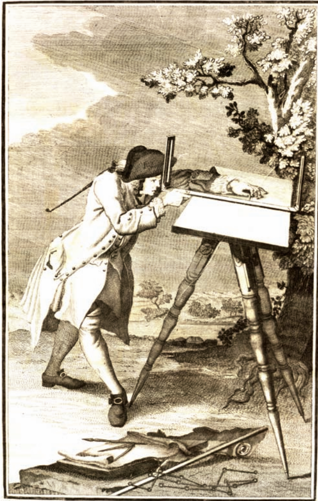
FIG. 818. SURVEYOR USING A PLANE TABLE. Johann Jakob Marinoni's book explained the details of using his tavola praetoriana , or plane table, in the process of surveying. From Marinoni, De re ichnographica (Vienna: Kaliwoda, 1751), plate facing page 10. Size of the original: 24.7 × 15.5 cm. Image courtesy of the Department of Special Collections, Memorial Library, University of Wisconsin–Madison.
