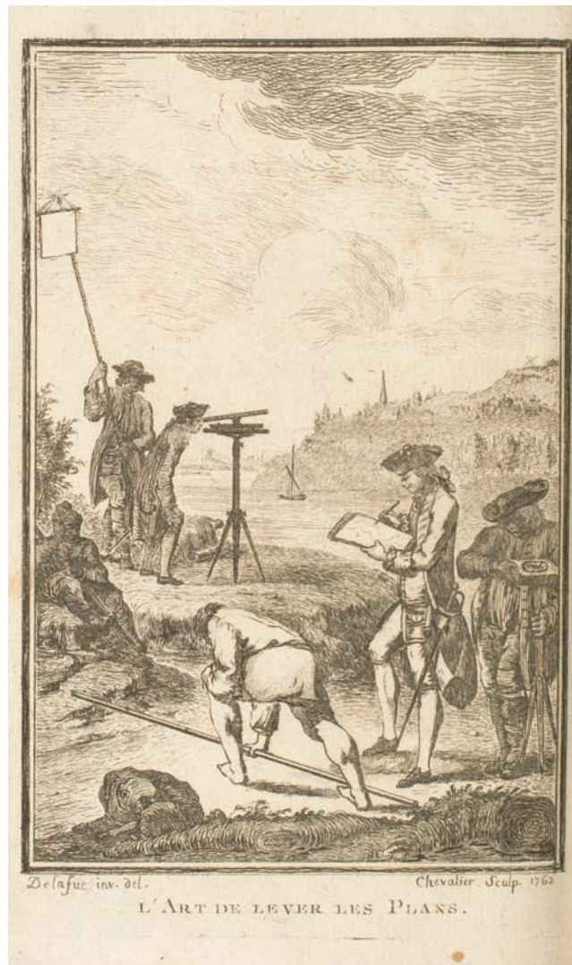
FIG. 817. SURVEYORS IN ACTION. The frontispiece to this popular textbook shows surveyors with plane table, sketch pad, measuring rod, theodolite, and sighting target. From Louis Charles Dupain de Montesson, L'art de lever les plans (Paris: Jombert, 1763).
