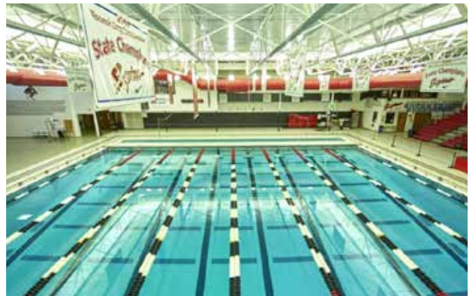
▲ A 2015 upgrade from metal halide lights to LEDs in Waukesha South High School's Natatorium provides safeguards against moisture and water treatment chemicals while reducing safety issues for lifeguards. Photo credit: Glen Norder, Waukesha.
