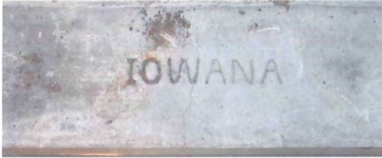
Figure 6. Top of concrete machine platform in Room D-3, with "IOWANA" etched in surface. Photo by Tallgrass Historians L.C., September 2010
