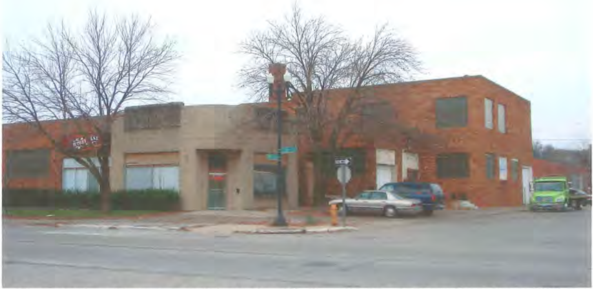
Figure 4. View of the Iowana building to the NW. Shows the SE entrance and two-story addition.
