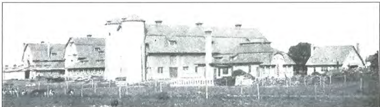
Figure 17. Photograph of Iowana Farms in 1914. French built his barns, outbuildings, and silos out of concrete, the recommended building material at the time for maintaining “absolute cleanliness”
