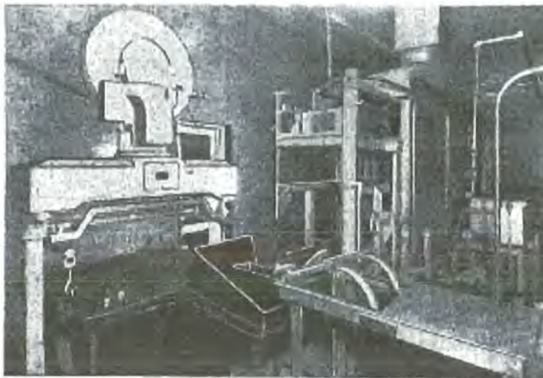
Protection from contamination of milk starts in the receiving room. The stainless steel suspended weigh can and straight-way can washer are designed to do just that.
