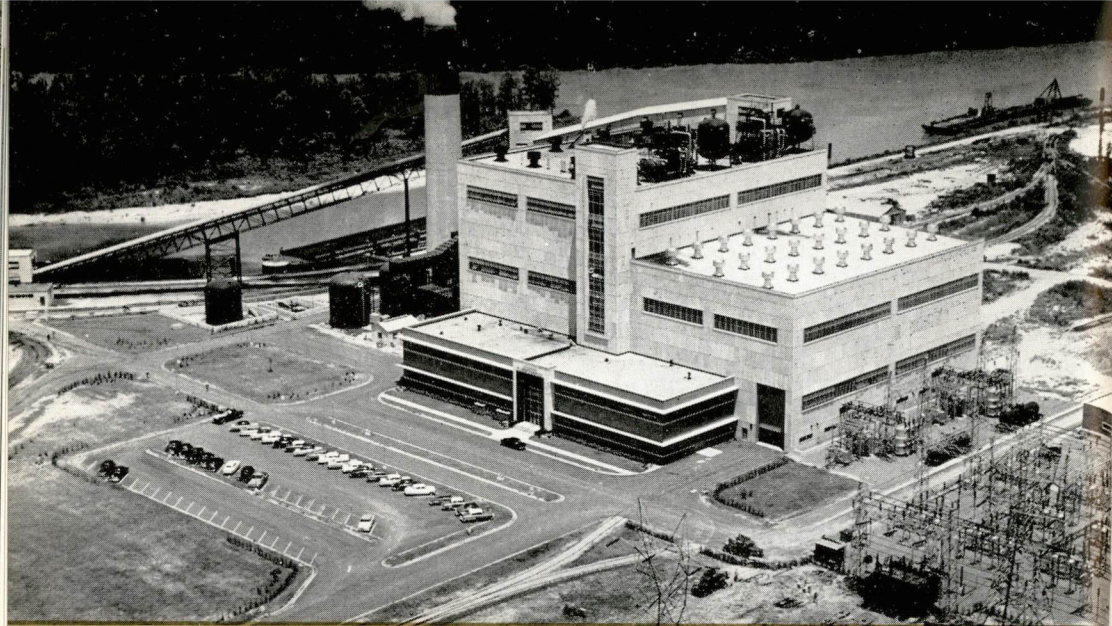
Barry Steam Plant, near Mobile, one of the most modern in the South
