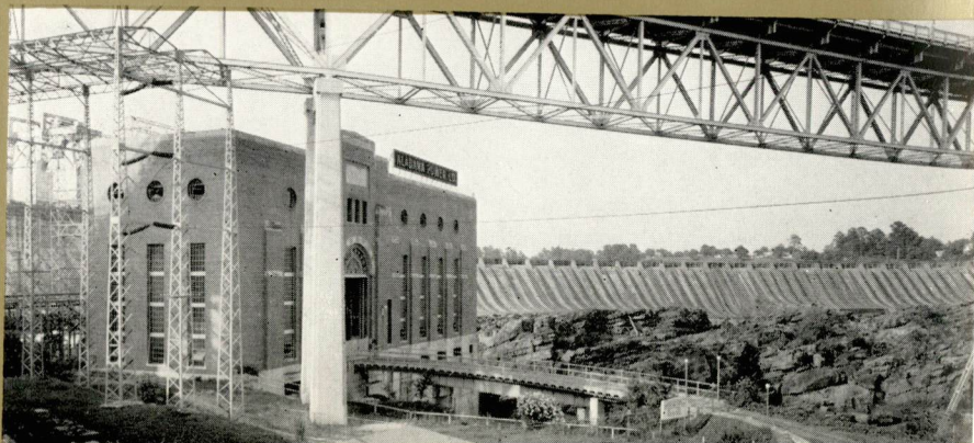
Thurlow Dam, at Tallassee, is one of the more picturesque in appearance. The low dam it displaced was a source of mechanical power for a number of years before the present generating plant was built.
