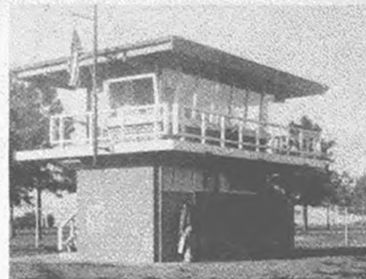
Two-level "control tower," one feature of the Charles A. Dannelly Modelport, in New Orleans.
