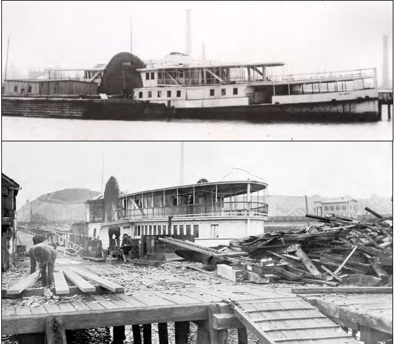
Figure 5-16. The Narragansett Bay excursion steamer Bay Queen (SW-18) at the Providence Dry Dock and Marine Railway Company dry dock pier in the process of being cut-down prior to its abandonment on the north side of the pier. These photos confirm the practice of the shipyard dismantling vessels for their valuable hardware or lumber prior to their disposal in the shallow waters of Green Jacket Shoal close to the dry dock pier and the marine railways (sources: William H. Ewen, Jr. Collection [upper image]; RIHS RHiX38351 [lower image]).
