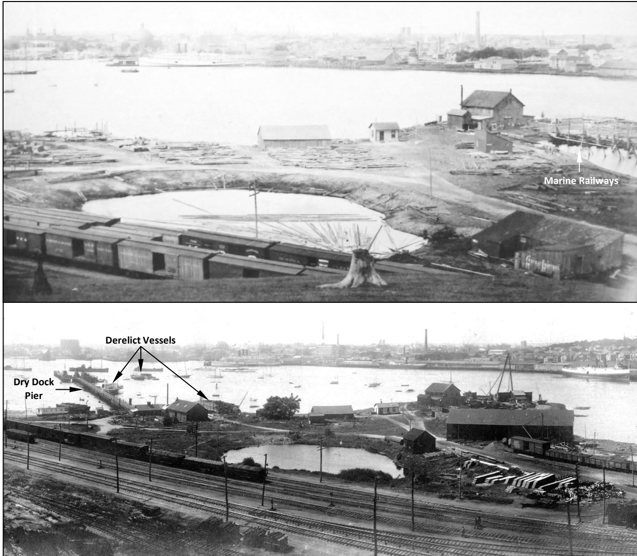
Figure 4-7. Two views of the Providence Dry Dock and Marine Railway Company's shipyard at Bold Point near the beginning and end of the yard's 35-year operational history. The upper photograph is from 1890, just six years after the business was established. It provides a partial view of the marine railways, several buildings, and a "timber-pickling" pond in the foreground. The lower image was taken by Archibald F. Ellis in 1910 after the company was in business for 26 years. The yard's infrastructure has been expanded with additional buildings and a rail spur visible on the property. Noteworthy are the absence of derelict vessels in the water or along shore in the 1890 image, and the presence of several derelict vessels in the 1910 image. This accumulation of derelict ships over the course of a 20-year period in the waters adjacent to the shipyard suggests a causal relationship between the vessel remains in the water today and the shipyard (source: Providence Public Library Rhode Island Collection [upper image]; Providence City Archives [lower image]).
