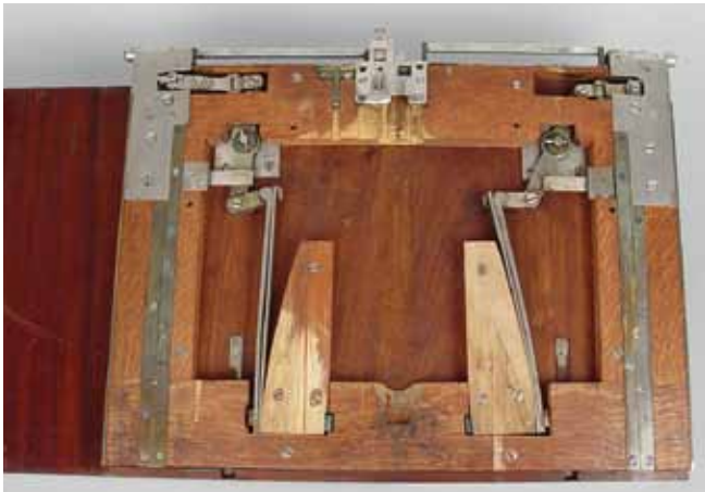
APP. 3.14. View of the underside of the folding desk showing the position of the springs and levers when one side panel is closed and the other open
