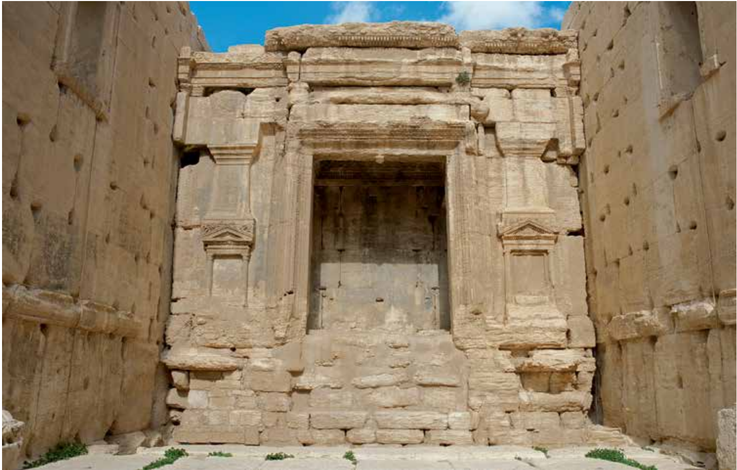
Fig. 57 Interior of north adyton of the Temple of Bel, Palmyra, prior to its destruction in 2015
