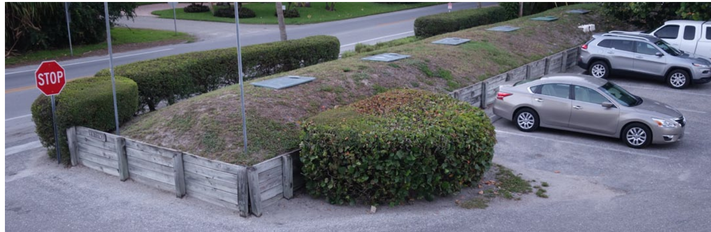
Septic tank mound, Captiva, FL.
