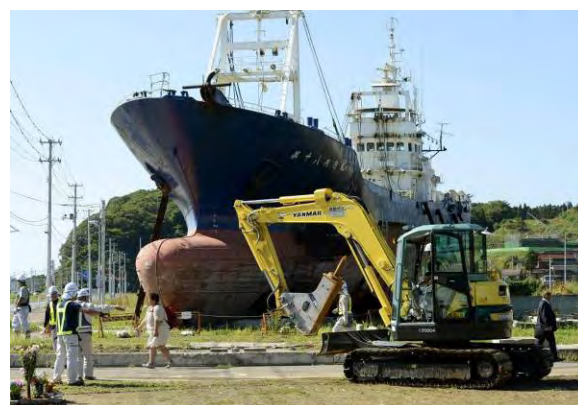
September 2013, work is starting © KYODO
