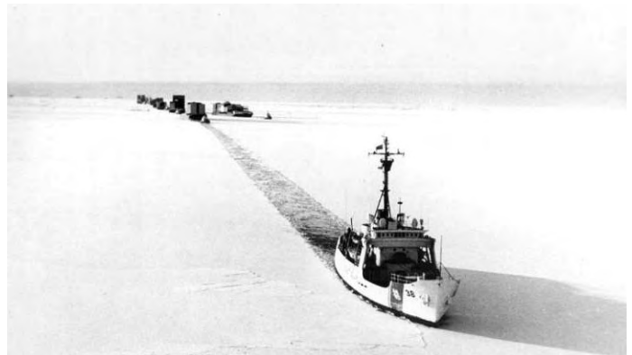
October 1 st , 1975, on the way to Prudhoe Bay
