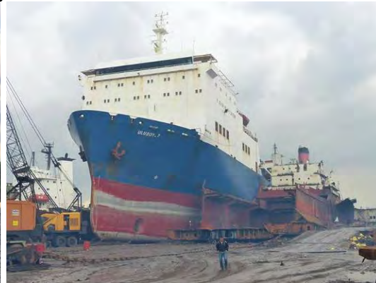
2013, Ulusoy 7 is beached for demolition in Aliaga (Turkey) © Ship Pax Information
