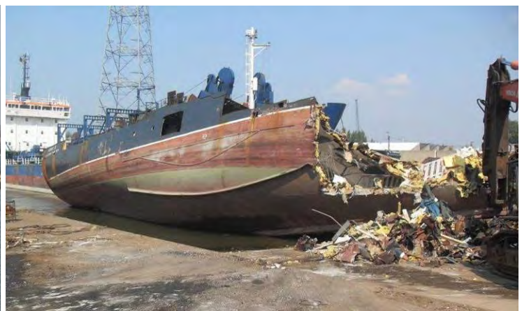
End of the demolition, September 4 th 2013 © Peter Wyntin
