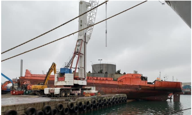
Copernicus , undergoing demolition in Grenaa (Denmark). © Leif Hansen
