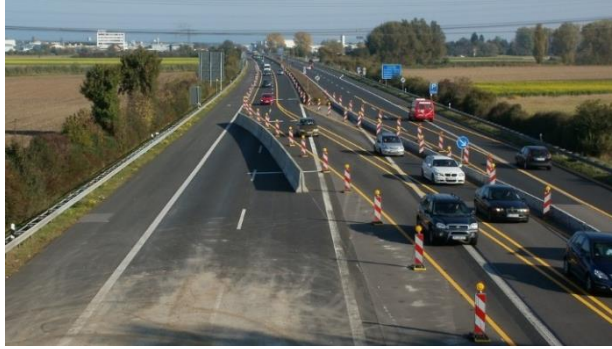
c. Temporary yellow markings at a crossover at an unspecified location on a German autobahn (2011)
