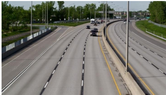
Figure 9. Black pavement marking used as a contrast color on Route 132 in La Prairie, Quebec
