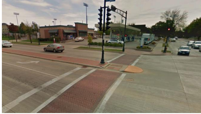
Figure 12. Simulated brick crosswalk and yellow marking used to increase median nose visibility in Shorewood, Wisconsin
