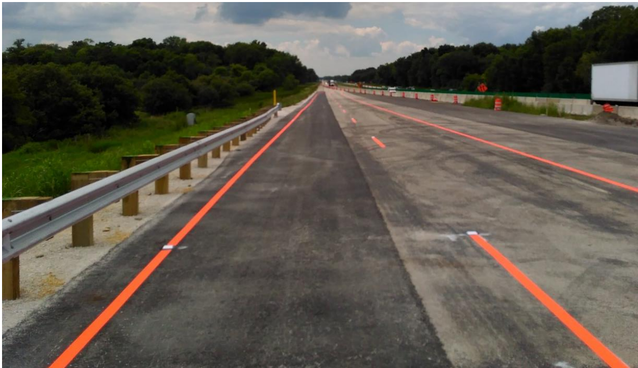
Figure 39. Freshly installed fluorescent orange pavement marking tape – Golden Lake Road – August 9, 2016
