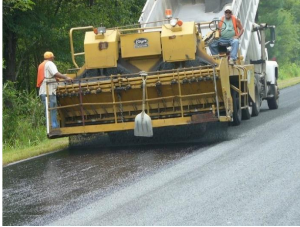
Figure 5. Chip seal application
