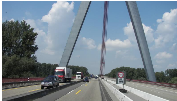
c. Temporary yellow markings at a crossover at an unspecified location on a German autobahn (2011)
