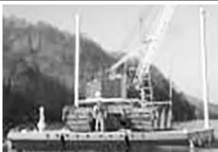
32' x 40' x 4' Sectional Spud Barge and Crane.
