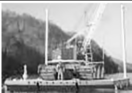
32' x 40' x 4' Sectional Spud Barge and Crane.
